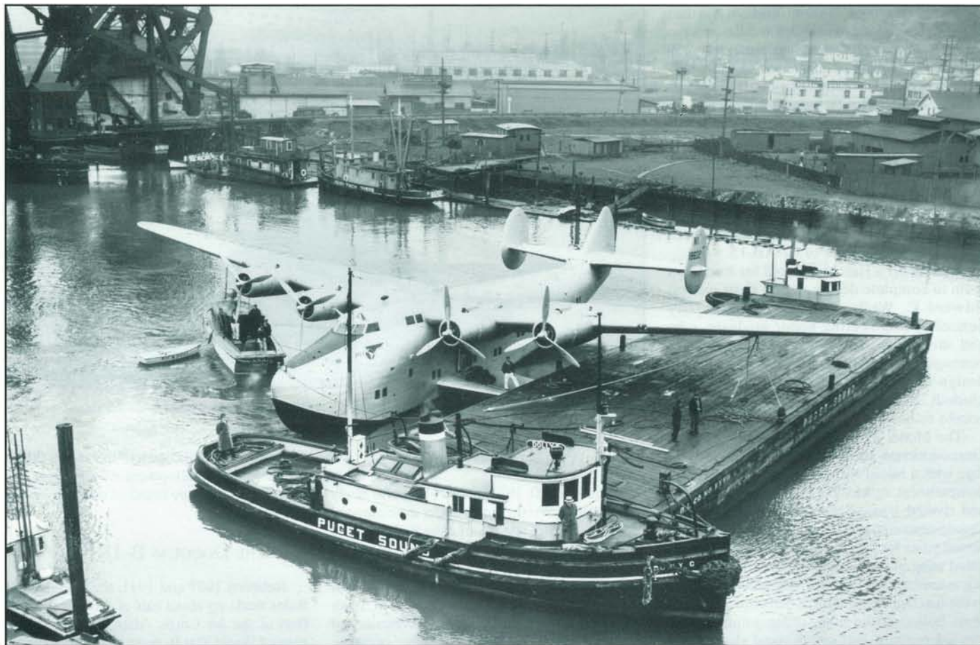
The XB-15 flew after the B-17, but its wing design, used in the B-17, had been proven earlier on the famed Model 314 flying boats purchased by Pan American World Airways and known as Clippers. This ship was the second in a series of 12 and still carried the experimental NX registry number on its tail. (Boeing Photo)
