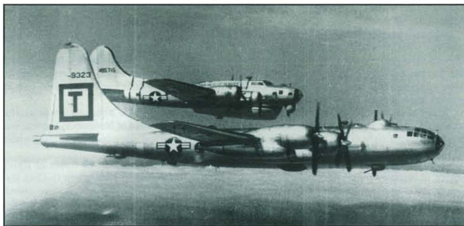
With the No. 2 and 3 engines pulling minimal power, Maj. Leman M. Herridge's crew managed to get this B-50D back to Lajes AB. A MATS Air Rescue Service SB-17G accompanied the laboring bomber. For their actions, they were selected as Crew of the Month by SAC's Combat Crew magazine. (Courtesy of M. Herridge)
