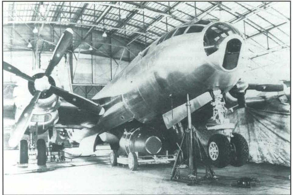
This B-50D had its nose raised on a jack to afford clearance for the loading of a Mk. 4 atomic bomb into the forward bomb bay. Note that the forward bomb bay door was also removed to permit clearance for the huge weapon. The aft bomb bay housed a fuel tank. (Courtesy of National Atomic Museum)
