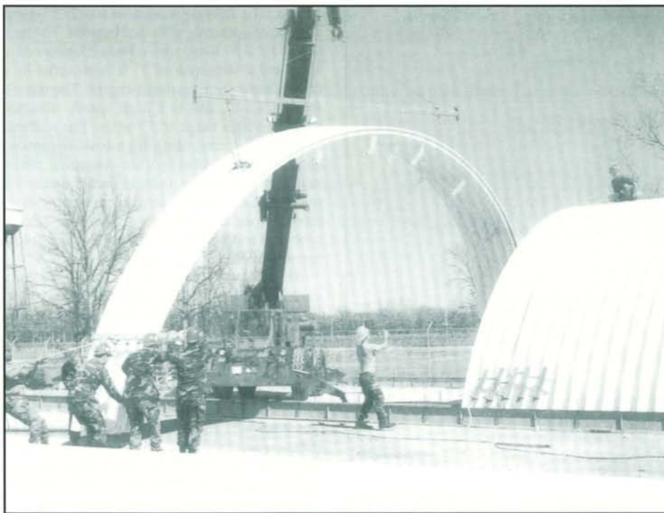
Members of the 2D Civil Engineering Squadron were practicing the erection of a temporary shelter. Such operations took place when Prime Beef Teams deployed in support of remote operations. (Courtesy of the United States Air Force)
